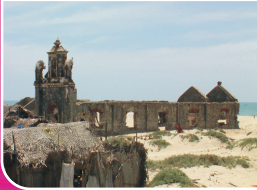
DHANUSHKODI CHURCH BUILDING
